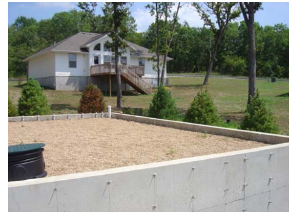
Residential wastewater treatment plant owned by Ozarks Clean Water Company.
